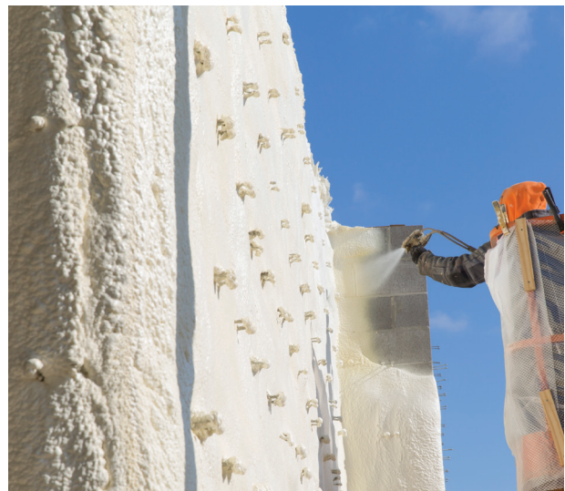
FIGURE 4. A cold weather exterior continuous insulation application of Icynene ProSeal Eco medium density spray foam in Michigan - November 2014.
